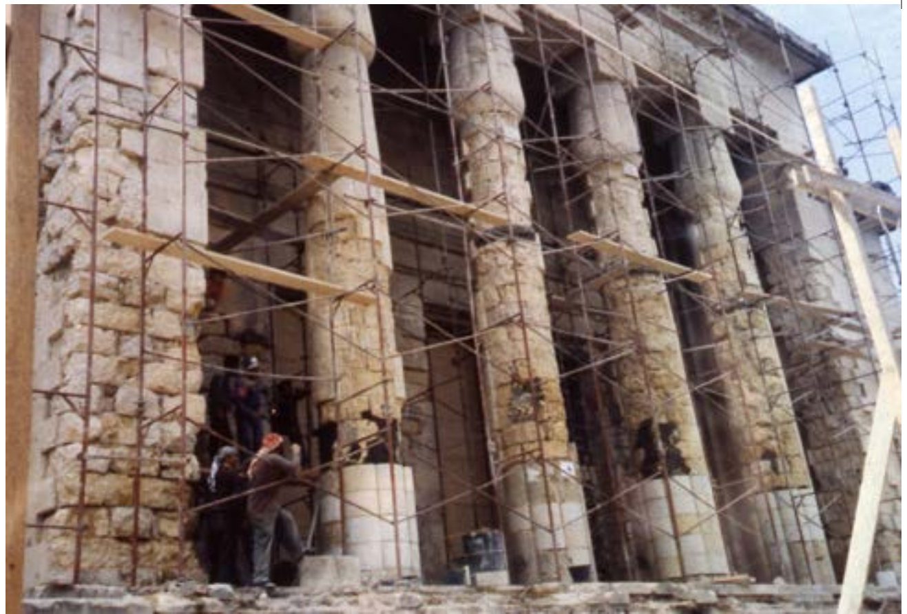
↑ Fig. 4: The Museum's main façade in 1996, during rehabilitation works, source: Farès el-Dahdah.
