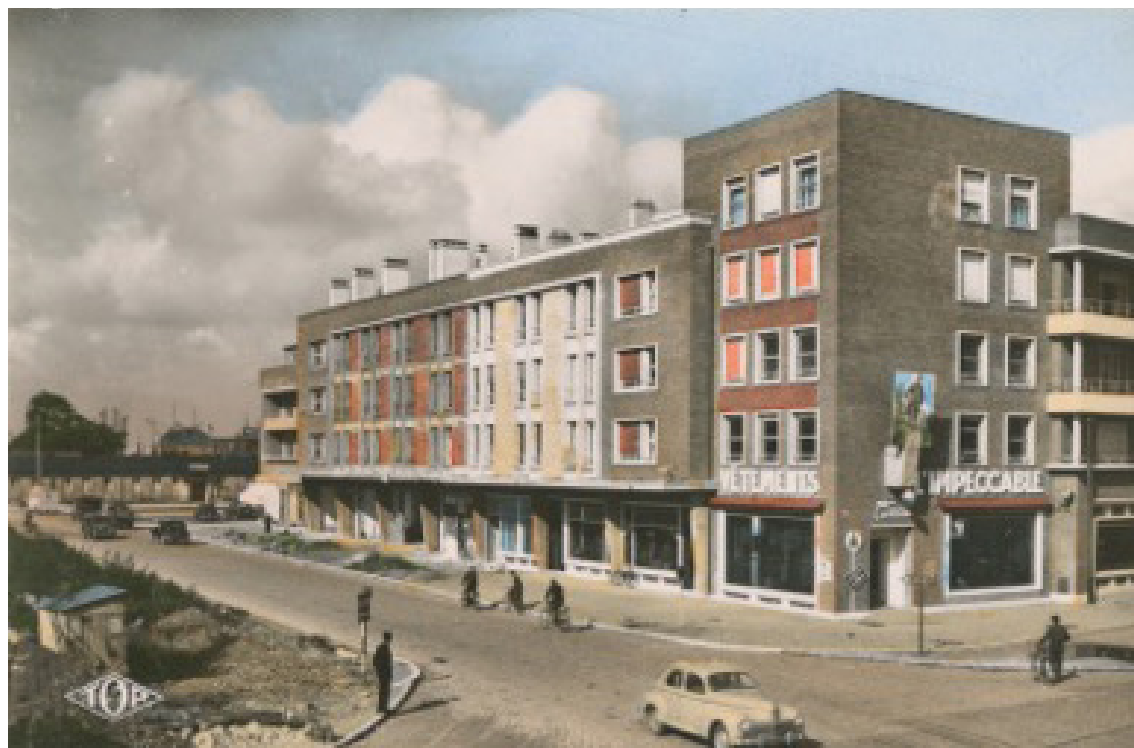
Fig. 5: Dunkerque, Rue de la Marine under reconstruction, source: CMUA.
